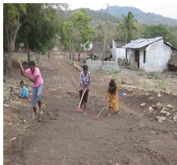
Side drain excavation and levelling in Covalima, Sub district, Maucatar, Suco: Ogues & Matae
