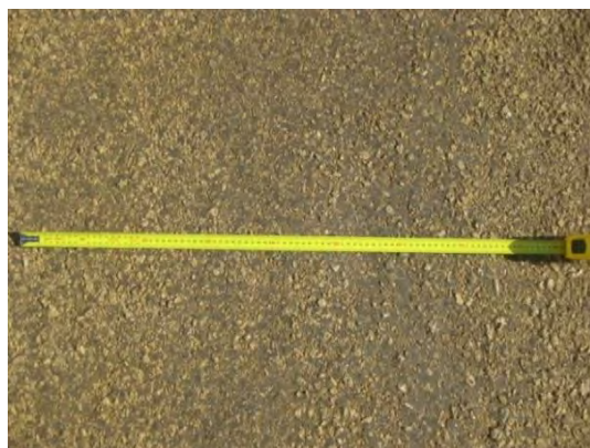
Figure 1 Pilot Otta Seal on Folaha Road with the best surface texture after 12 months of traffic
