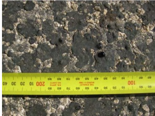
Figure 2 Excess bitumen at Fonongahina Road and Liku Road intersection
