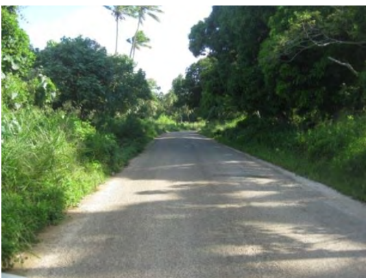
Figure 1 Pilot Otta Seal on Folaha Road with the best surface texture after 12 months of traffic
