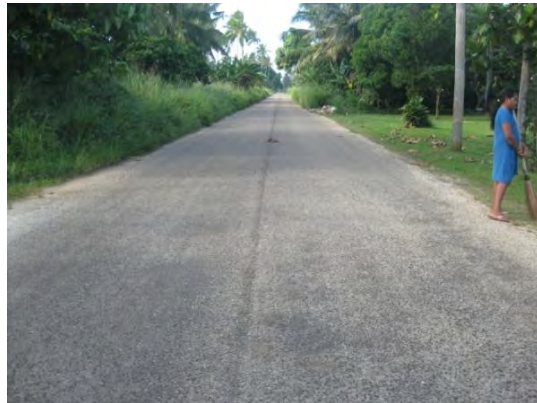
Figure 3 Stop-Start (Transverse) Joint Holoipepe Rd and Seal overlap at middle – Folaha Rd
