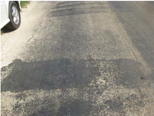
Figure 3 Stop-Start (Transverse) Joint Holoipepe Rd and Seal overlap at middle – Folaha Rd
