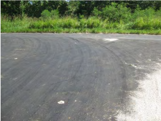
Figure 2 Excess bitumen at Fonongahina Road and Liku Road intersection
