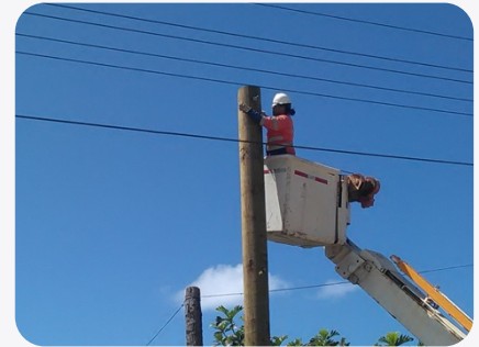
Female line technicians install new wirings on 'Eua
