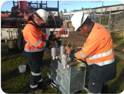
Wiring new transformers on 'Eua
