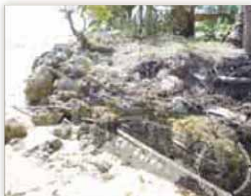
Photo 7: Coastal erosion in Manuka Village, 2006.
