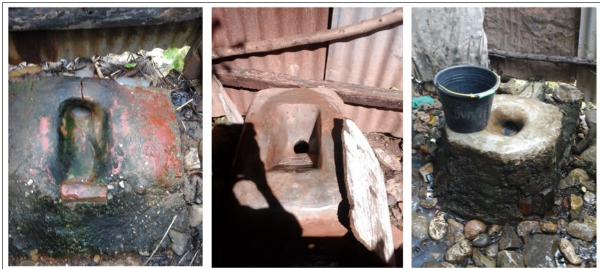
Figure 12. Type of cement toilet pan/bowl observed (self-made by households)
