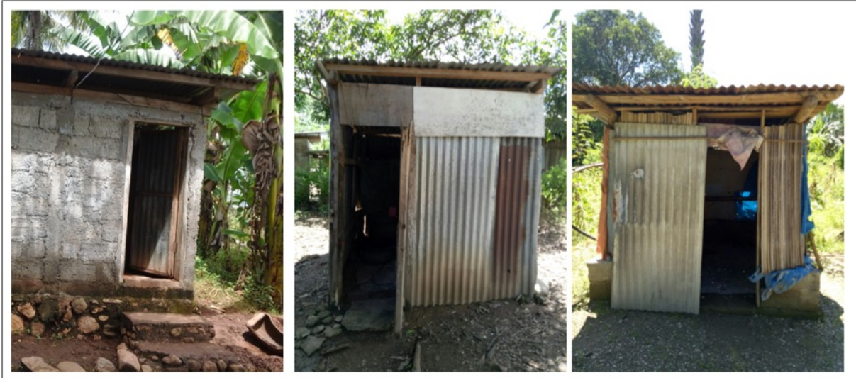
Figure 14. Type of toilet wall/superstructure observed (concrete(left), corrugated zinc sheets (middle) and combination of babak and corrugated zinc sheets (right)
