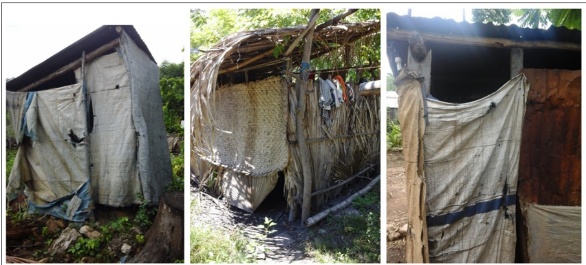
Figure 15. Type of toilet wall/superstructure observed (terpal (left), palm leaves (middle), and combination of terpal and corrugated zinc sheets (right)
