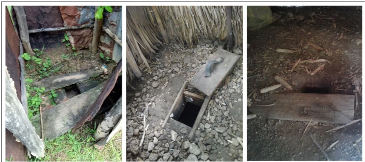
Figure 8. Pit latrine without slab/open pit observed
