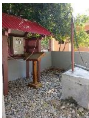
The covered well and pump, and the electrical control box.
