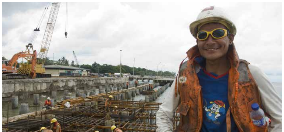
Port construction in Dili, 2008. Photo: Lorrie Graham, DFAT
