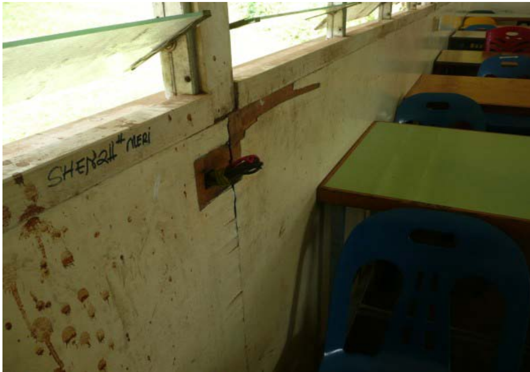
Dangerous exposed wiring. Buai spit on walls and floor
