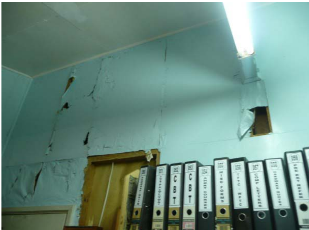
Termite damage in teacher's office
