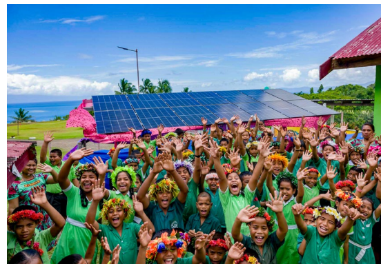
Primary students in front of newly installed solar panels at their school on Fiji’s remote Rabi Island. Credit: DFAT/AIFFP
