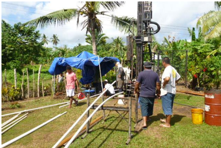
Figure 10: Monitoring borehole drilling and installation at Faleasiu.
