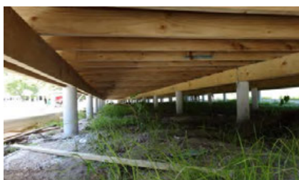
St John Bosco PS - single storey kitset with raised timber floors
