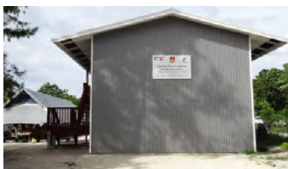
St John Bosco PS - single storey kitset with raised timber floors
