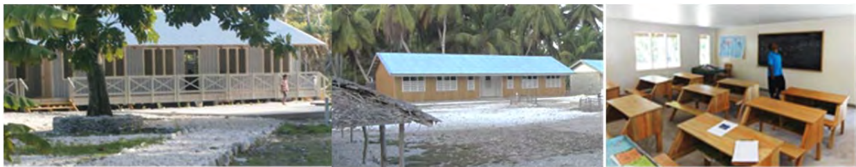
New kitset classrooms raised on timber stumps – Teeraka PS, Butaritari (2012)
