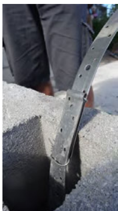
Stainless steel strap reinforcing
