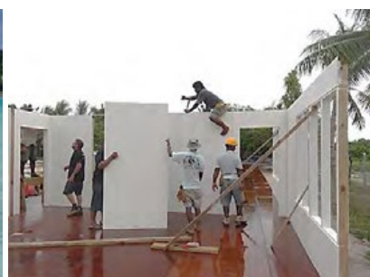
Kitset classroom block under construction at Bareaumai PS
