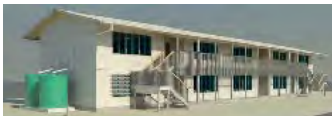
Rurubao PS - two storey 8 classroom kitset on a concrete slab
