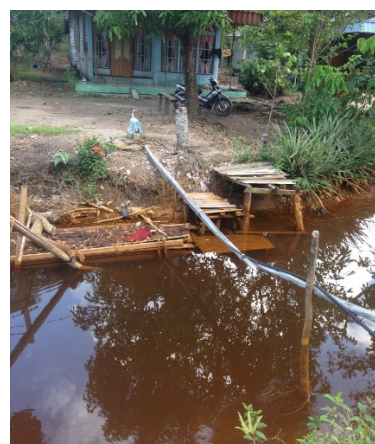
Figure 7: Insecure piping crossing waterway
