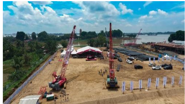
Figure 1: The Palembang wastewater treatment plant under construction in January 2021
