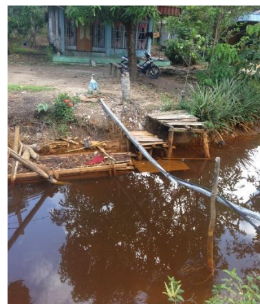
Figure 7: Insecure piping crossing waterway
