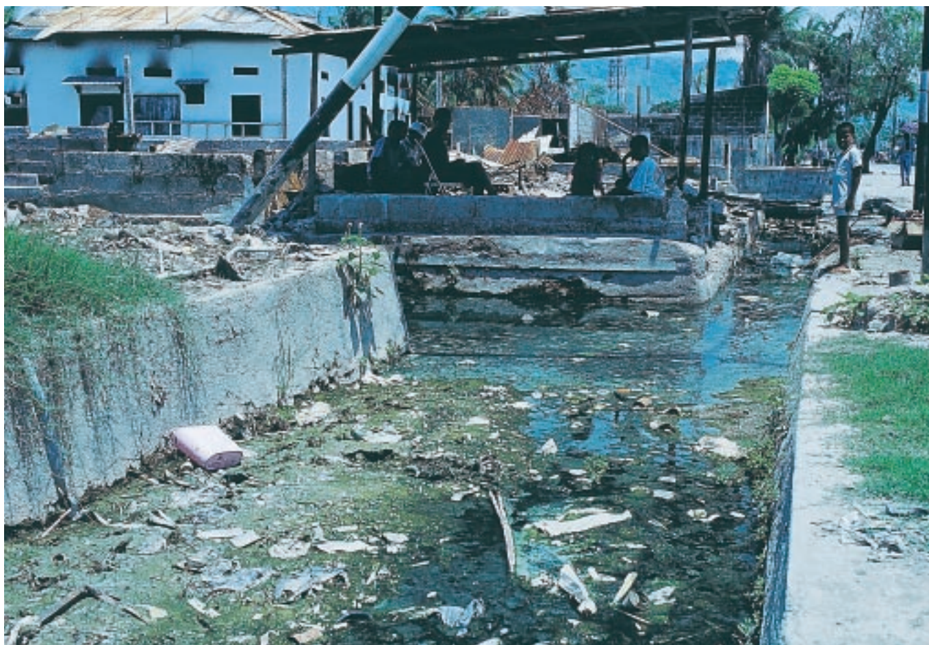
Blocked drains in Dili cause flooding and health problems.
