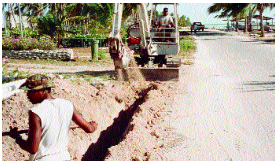
Locally employed workers dig trenches for water pipes to be laid in the town of London, Kiritimati (Christmas) Island, in February. Aimed at improving health on the island, the project is funded by the Australian Government. Photo: Doug Melvin
