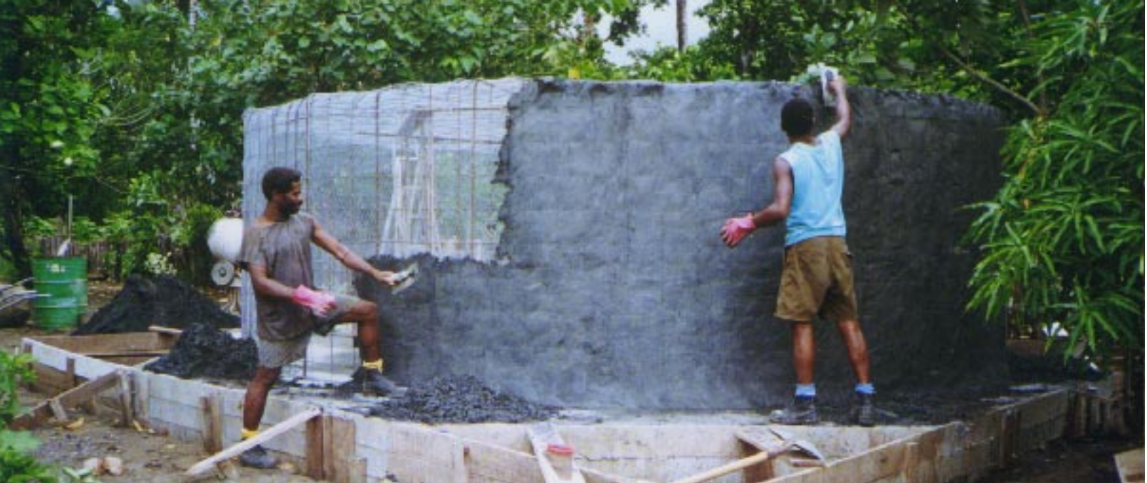
2. Laying the first of 8 layers of concrete over the frame of a 10 000 gallon ferro-cement tank near Gloucester
