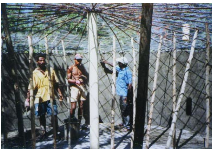
4. The inside of a 10 000 gallon ferro-cement tank following application of the last of 8 layers of cement to the wall Photo: P Cosgrove
