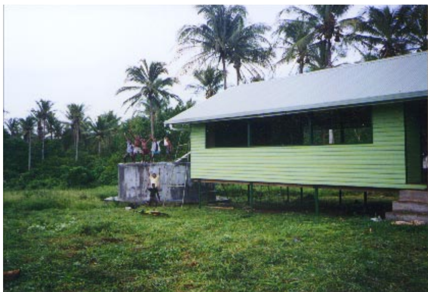
6. A near-complete 10 000 gallon ferro cement tank for the double classroom at Cape Gloucester
