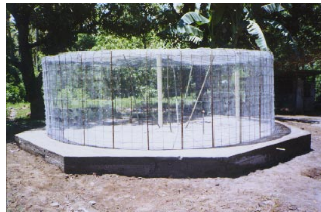
1. The initial structure for a 10 000 gallon ferro-cement tank after completion of the base and frame
