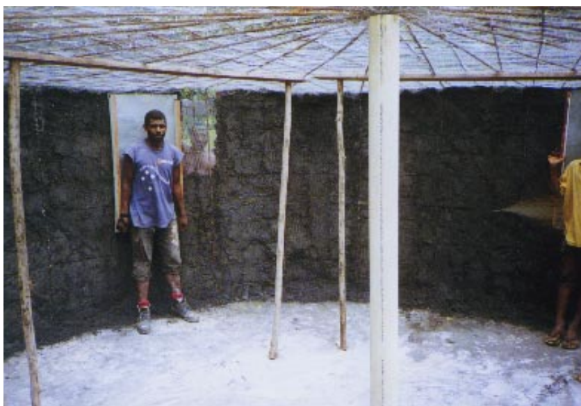
3. The inside of a 10 000 gallon ferro-cement tank during application of the 1st of 8 layers of cement Photo: P Cosgrove
