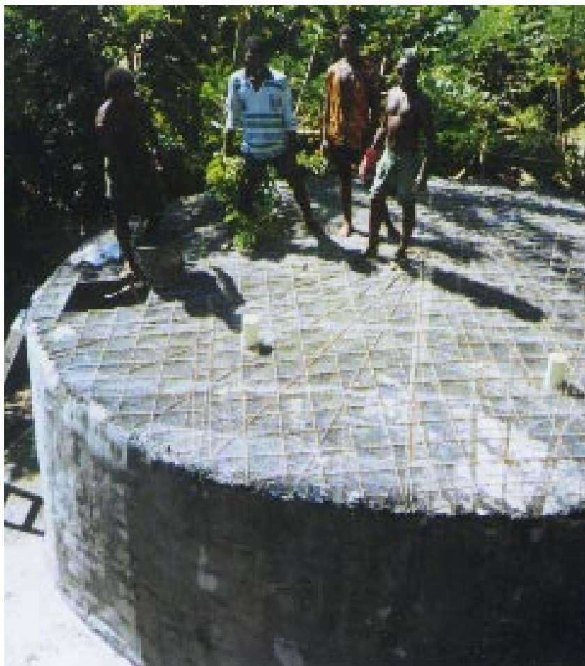
5. Testing the strength of the roof on a 10 000 gallon ferro-cement tank following application of the first few of 8 layers of cement
