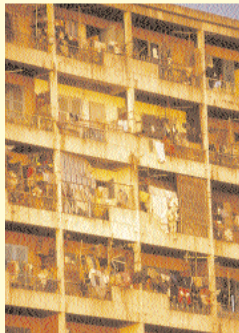
Inner city housing in Hanoi.
