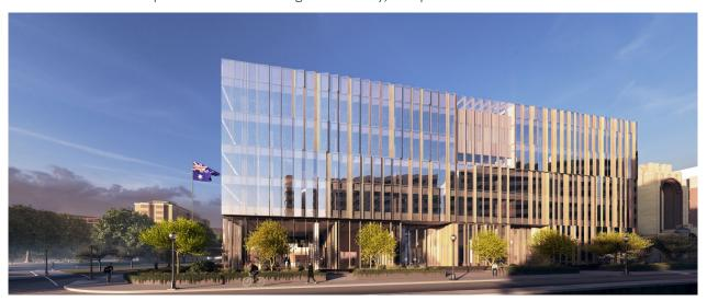
The new Embassy building includes a thermally efficient façade, a green roof with an extensive photovoltaic array, the expansive use of natural light, and the latest building services technologies. It also hosts a rooftop apiary, which can serve as home to approximately 240,000 resident bees.
