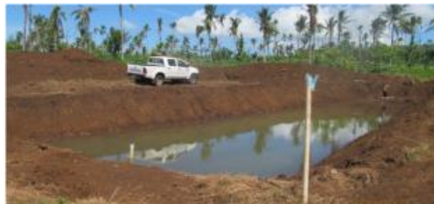
A view of one of the two new tilapia earth ponds dug by the excavator. The ponds are gravity fed and drained so there is no need for electrical water pumps.
