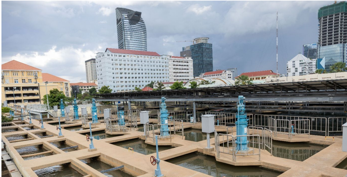
Photo: Phnom Penh Water Supply Authority's water treatment plant, CAPRED 2025
