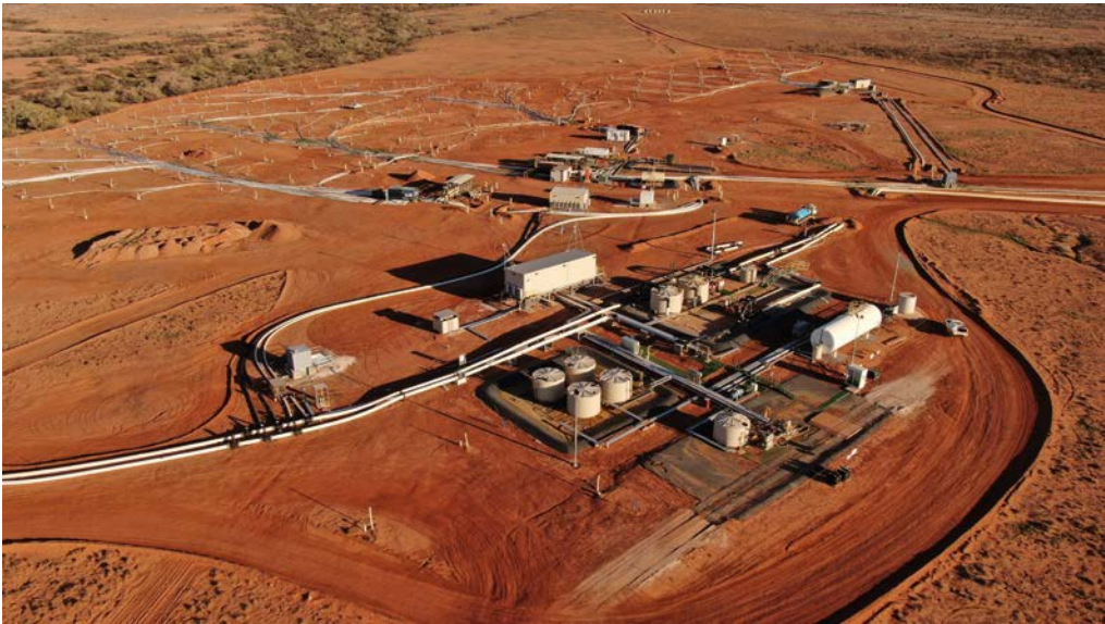
Booster and degas station with wellfields in the distance, at the Beverley uranium mine (Credit: Heathgate Resources).
