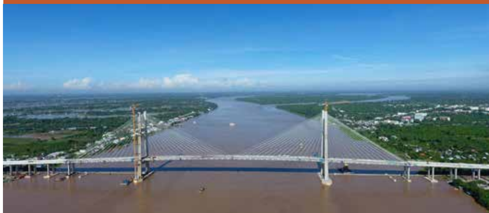
Cao Lanh Bridge, Vietnam. Photo: DFAT
