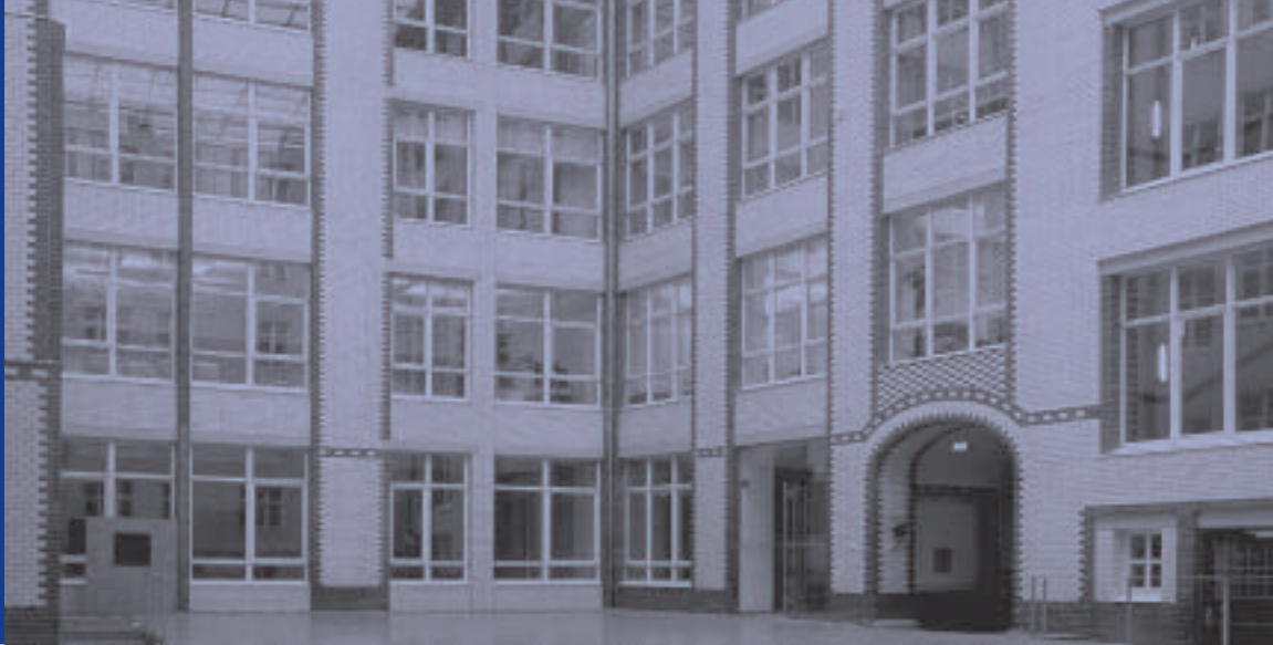
The internal courtyard of the new Australian embassy in Berlin. The building of the chancery was one of the department's most significant construction projects. The embassy was officially opened by the Minister for Foreign Affairs, Mr Alexander Downer, in January 2003.
